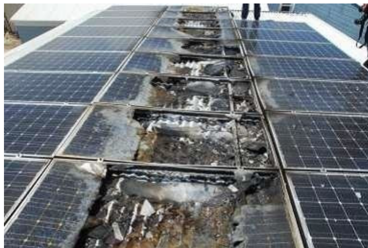
Figure 1: Arc Fault in a Solar Power System
