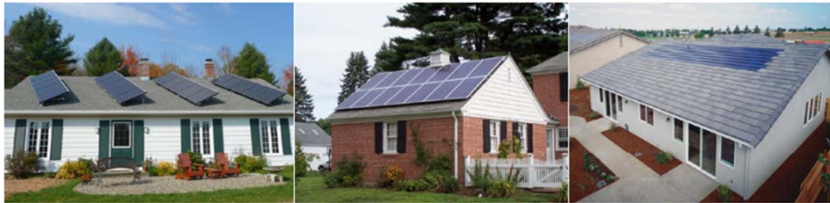
Figure 3: Examples of increasing integration of PV Panels [14]
