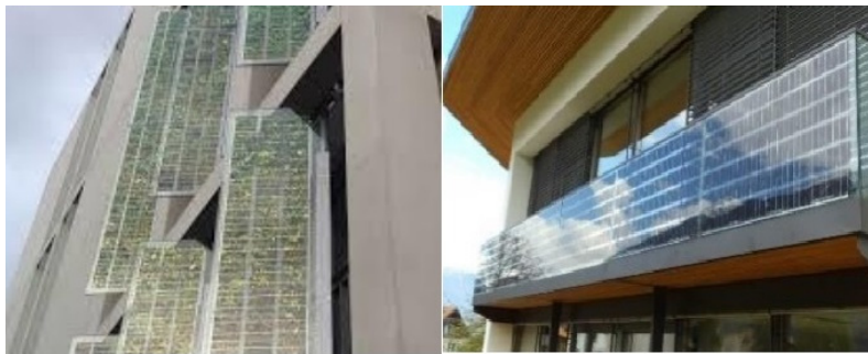
Figure 8: BIPV systems on external integrated devices [20]
